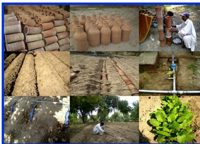
Figure 1. Baked clay pipes and their installation at the experimental field.
